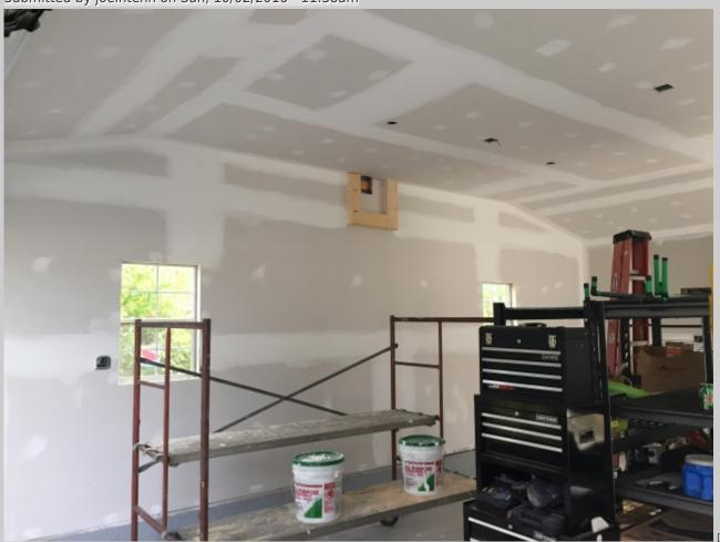
The drywall is finished. We are waiting on the painter, the electrical to be finished, then the garage floor to be resurfaced.
